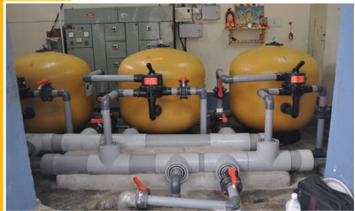
Swimming pool machinery of purification of water in the pool.
